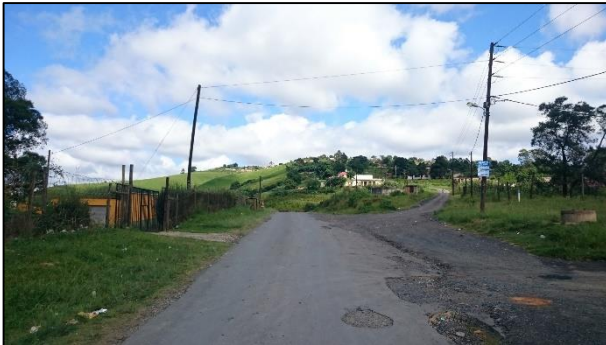
PLATE 21: Deteriorating road. Surrounding landuse is informal housing and subsistence agriculture.
