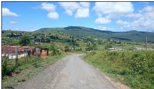
PLATE 2: Deteriorating road surface.
