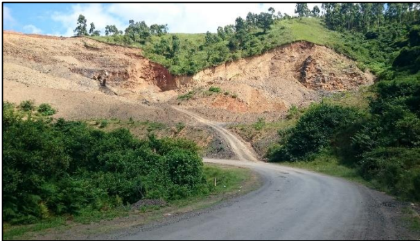
PLATE 9: Road surface in vicinity of borrow pit. There is a watercourse crossing draining from right to left at the bend in the road.
