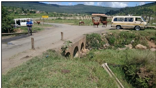
PLATE 1: Bridge at start of road upgrade project (chainage 0.0 km).
