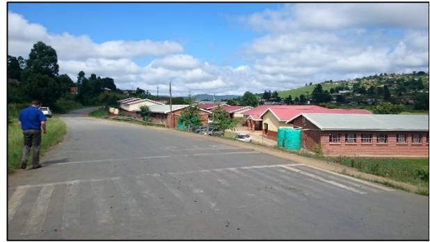
Plate 26: End of road upgrade project (chainage 4.3 km). A culvert drains from left to right beneath the zebra crossing.
