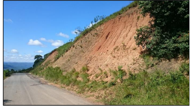
PLATE 124: Eroded cutting.
