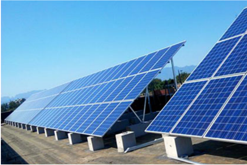
Figure 6: Visual of structures
