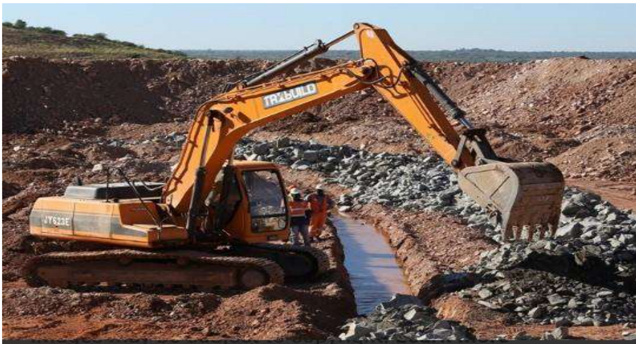
Figure 4.2: Illustration of dirty water trench
