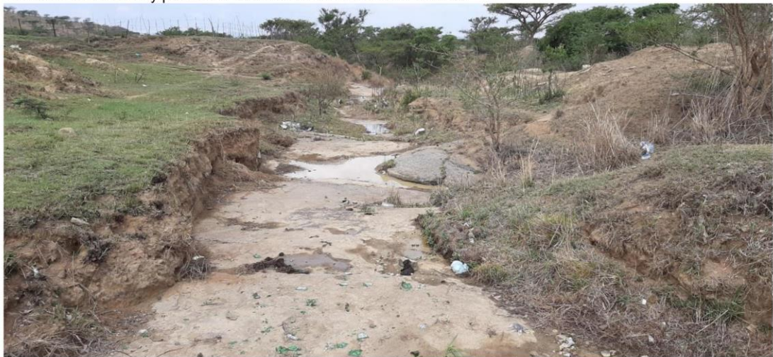
Photo 18: Bedrock controlled section of River Unit R2-A.
