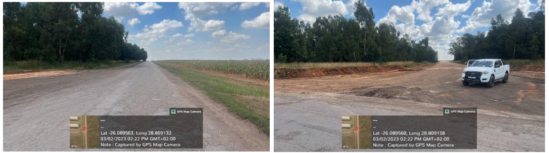
Figure 11: access road to site
