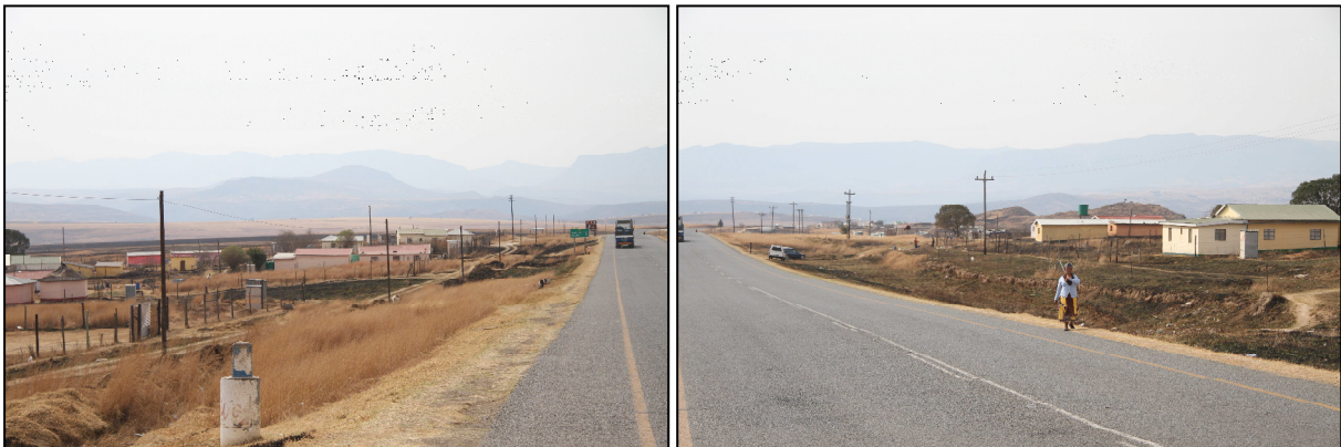
Plate 3: Photos indicating the types of structures occurring along the road route proposed for upgrade and rehabilitation.
