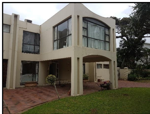
Plate 2: Front view and main entrance of the existing residential dwelling.
