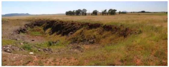
Figure 2: Panorama of the site showing the existing borrow pit excavation. Note that it remains free draining.
