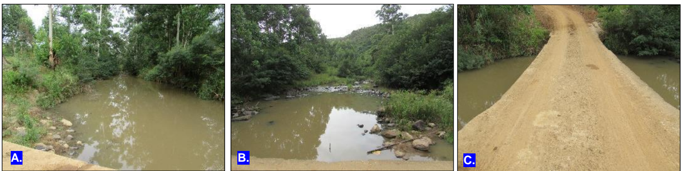
(a): Image upstream of RC97 (b): Image downstream of RC97 (c): Image showing the structure crossing the Mzimkhulwana River, to which the pipeline will be tied onto.
