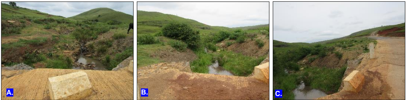
(a): Image upstream of RC59 (b): Image downstream of RC59 (c): Image showing the structure crossing the Nkondwana River, to which the pipeline will be tied onto.
