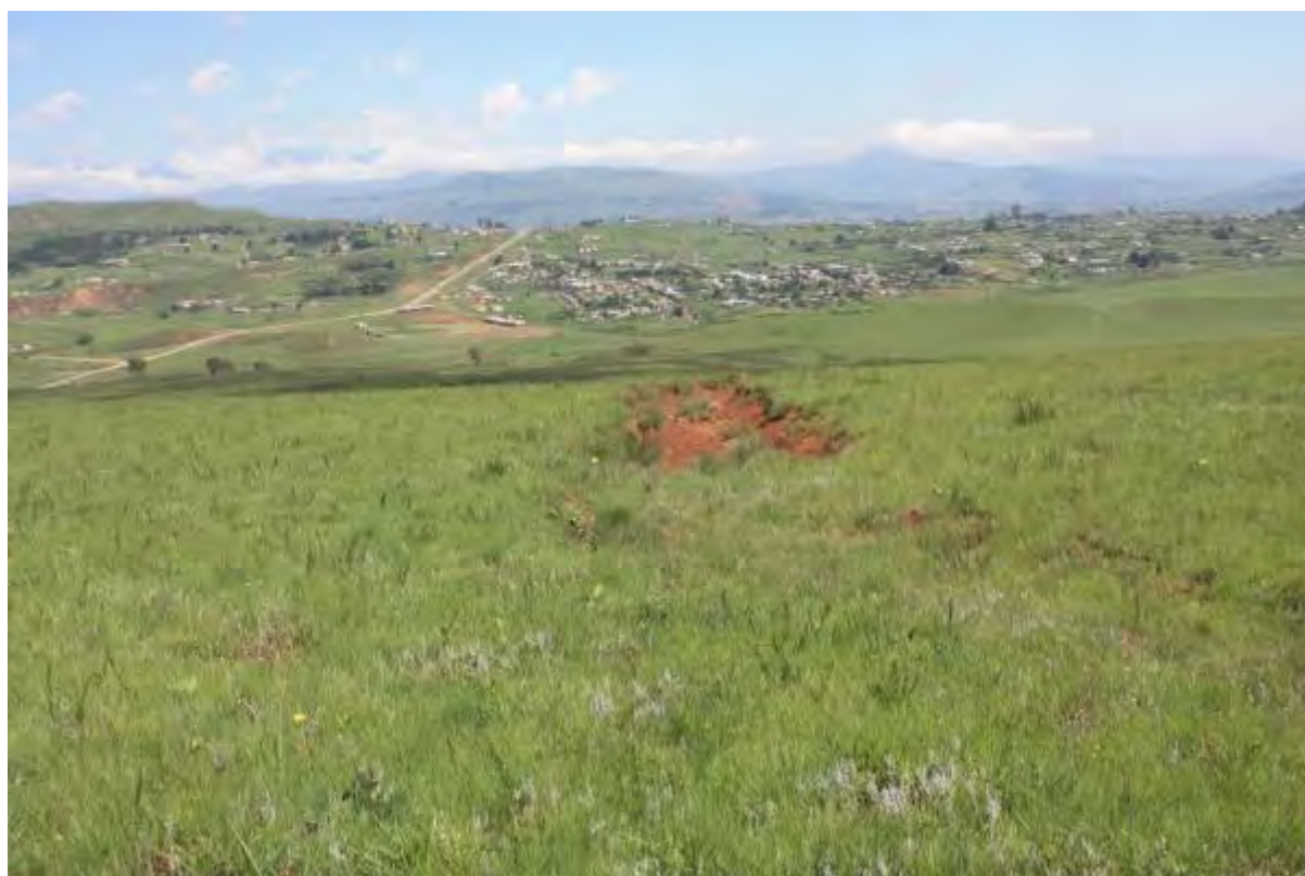
Fig. 9 Image of site indicating erosion gully arising where vegetation cover is reduced
