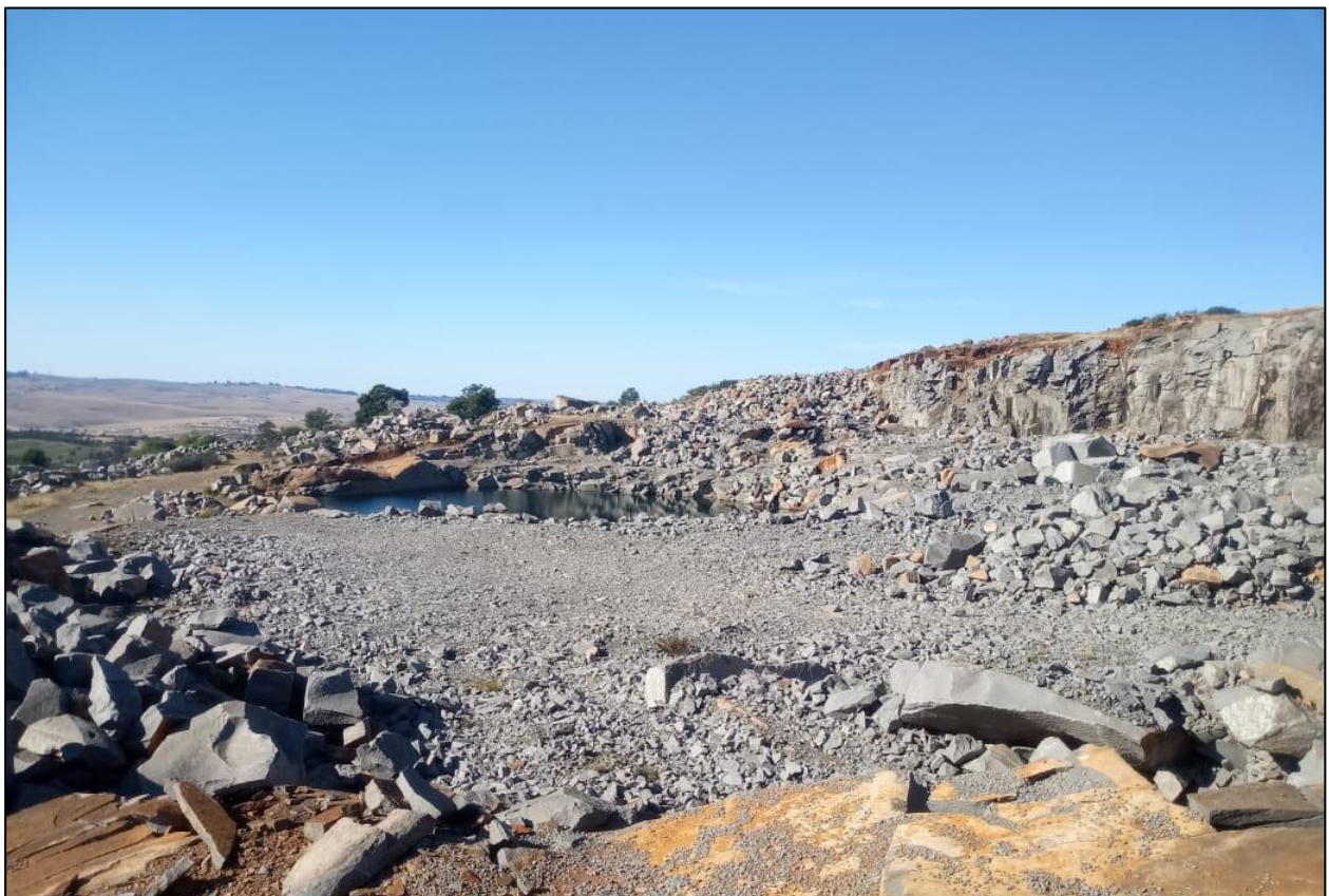
Photo 1: The existing highwall and pit floor of the old Laman Quarry from which mining will resume and where the mobile crusher will be placed.
