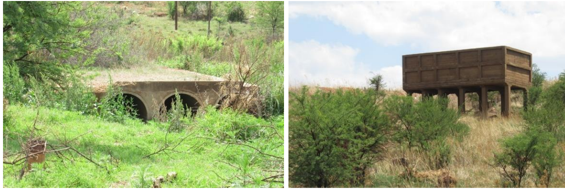
Concrete road bridge
