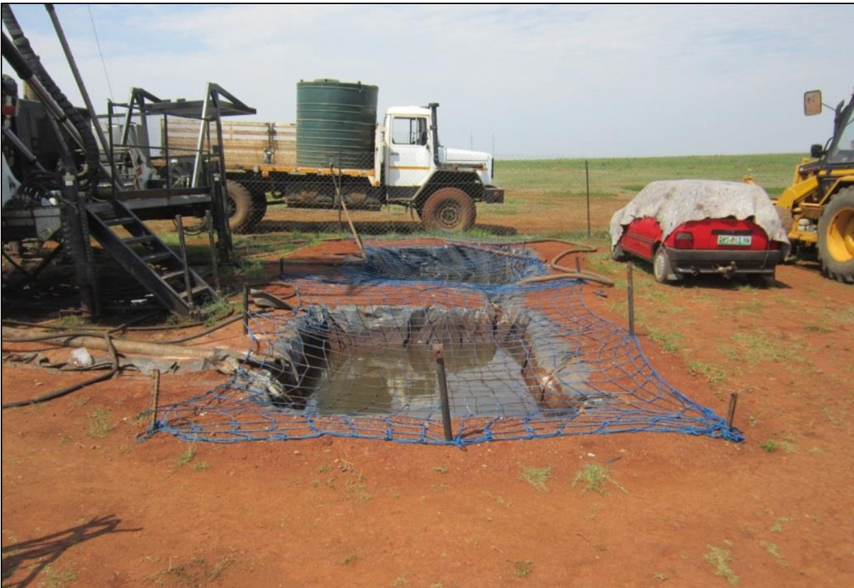
Photograph 2: Indication of the sumps required for a typical drilling operation.
