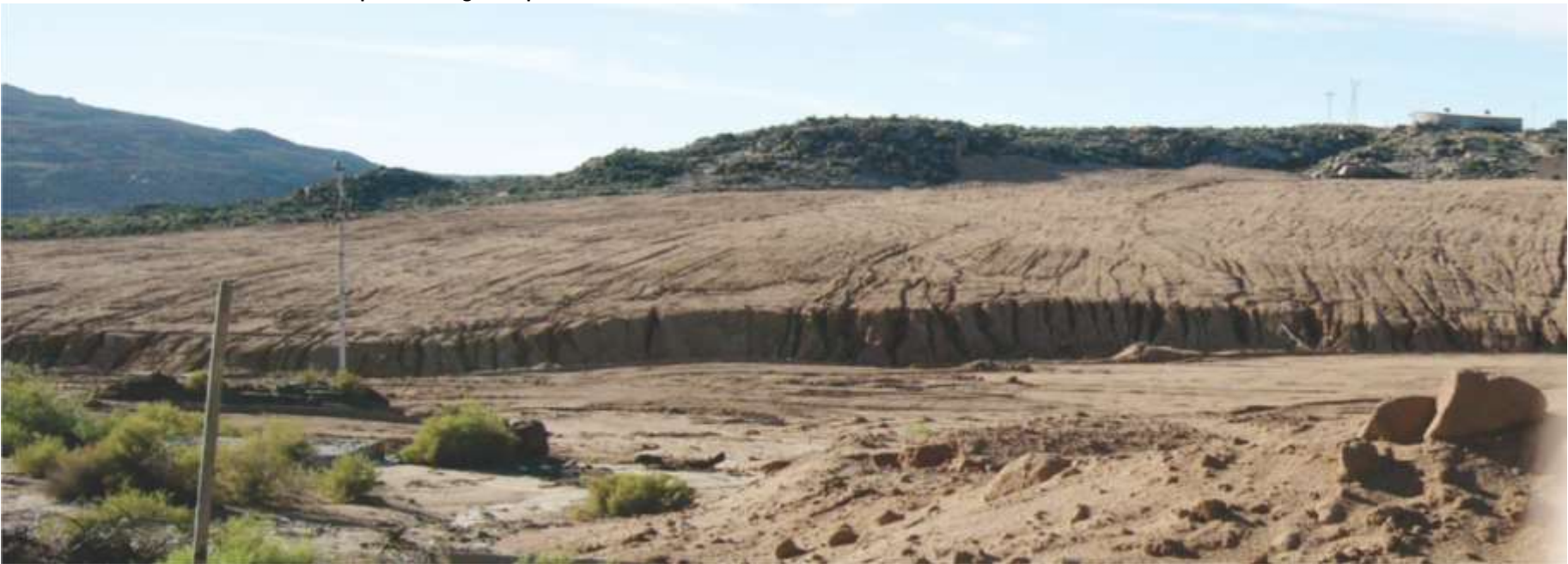
Photo 2: The Carolusberg leachate dump from higher lying area to the north. Note that this photo was taken in 2005 and the site looks better than this with less erosion and some revegetation in the foreground
