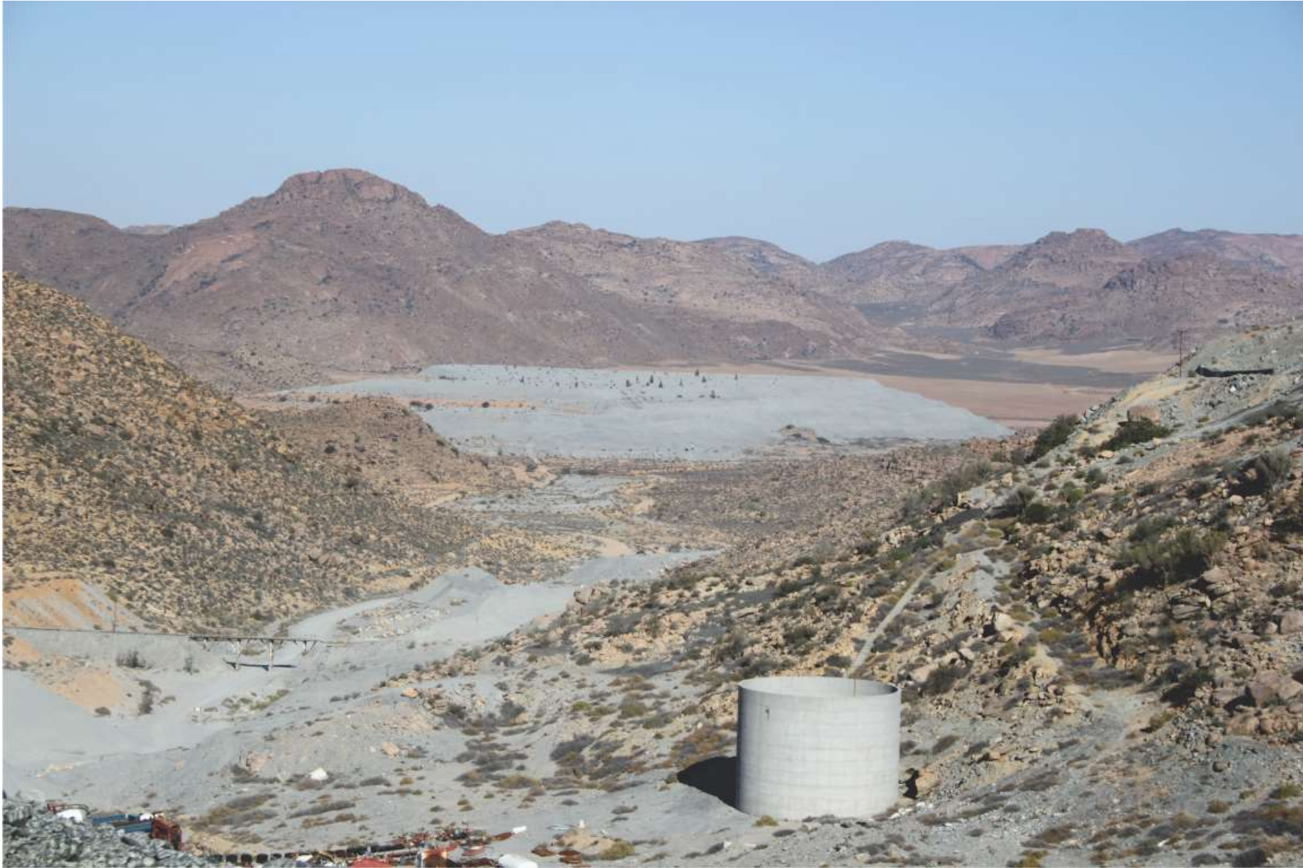
Photo 3: Distant view of the Carolusberg Fine Tailings Dump from the hill to the north overlooking one of the concrete capped shafts in the foreground
