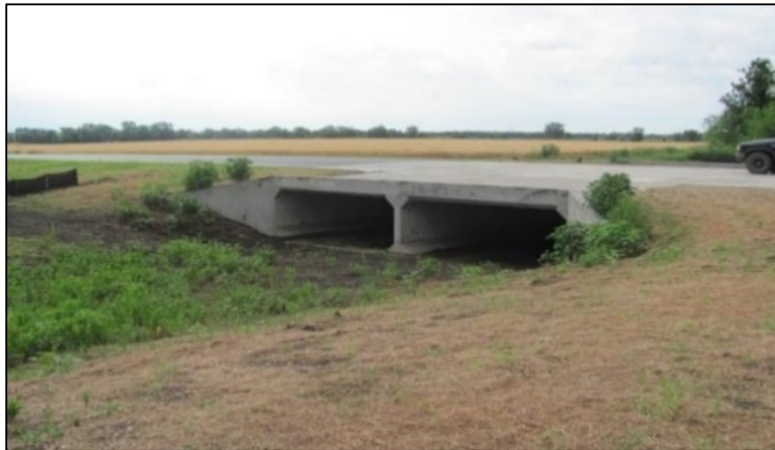
PLATE 4-2: Example of box culvert bridge crossing
