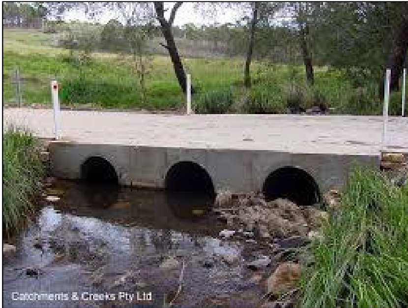
FIGURE 7-9: Example of pipe culvert crossing in a watercourse
