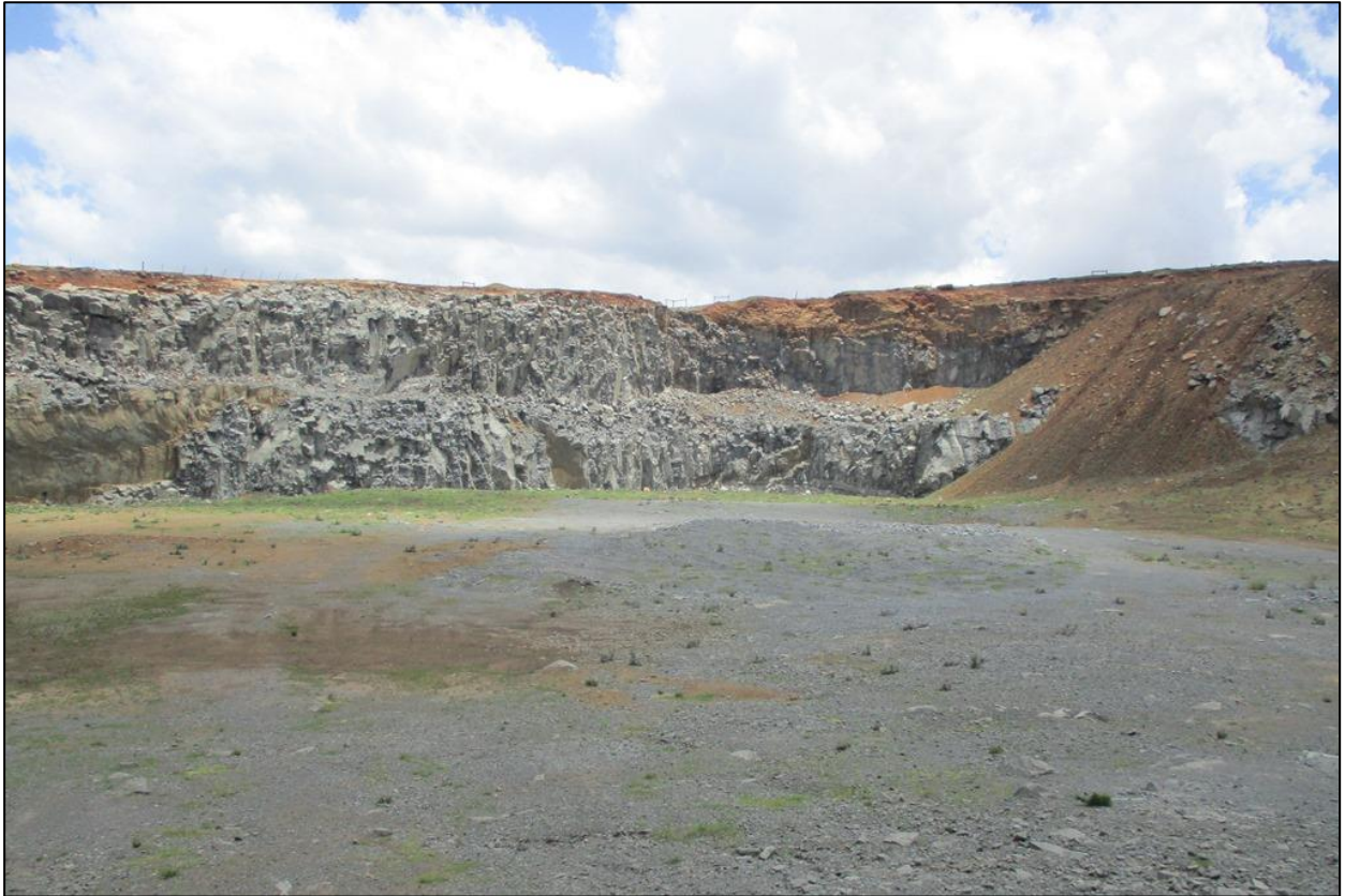
Photo 1: The existing highwall and pit floor of the old Yomba Quarry from which mining will resume and where the mobile crusher will be placed (Nicholson, Dec 2020).
