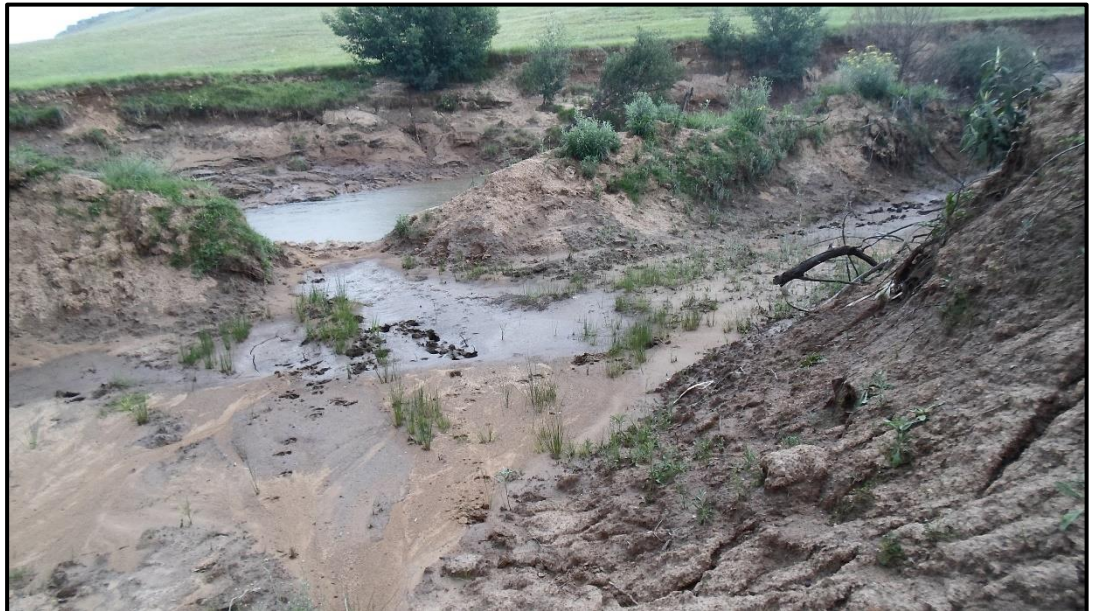
Figure 33: Photograph of the observed instream alterations of the Tsitsa River – November 2022 (Image obtained from the ABSA)
