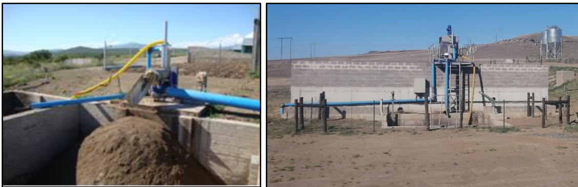
Figure 1: Images portraying a screw press system to be utilized on site
