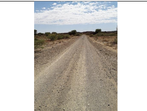
EXISTING ROAD INFRASTRUCTURE
