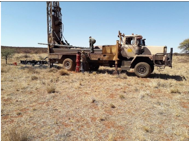
PERCUSSION DRILLING OF A BOREHOLE
