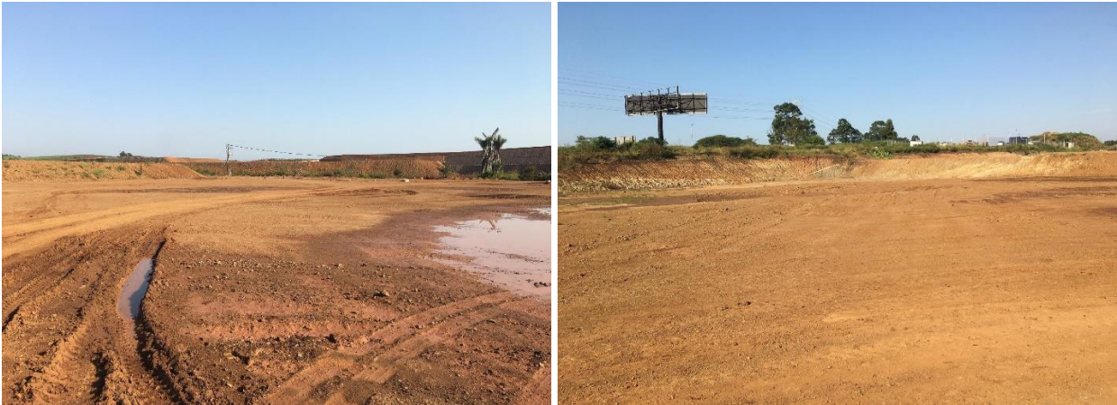
Figure 6 and 7: Aspect of the cut to fill site following bulk earthworks.
