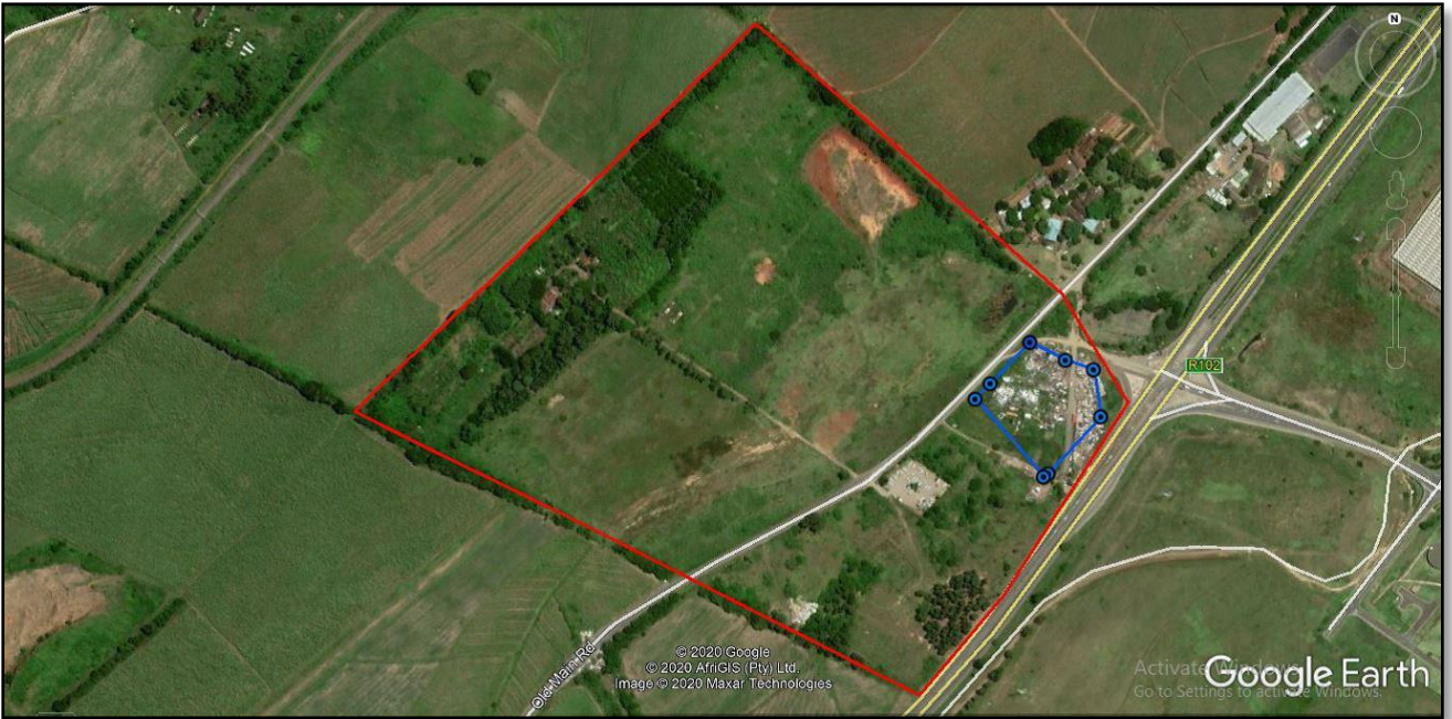
Figure 4: Approximate extent of Whetstone Development (outlined in red) with extent of Portion 8 (of 1) Erf 147 Mount Moreland at south eastern corner (outlined in blue).
