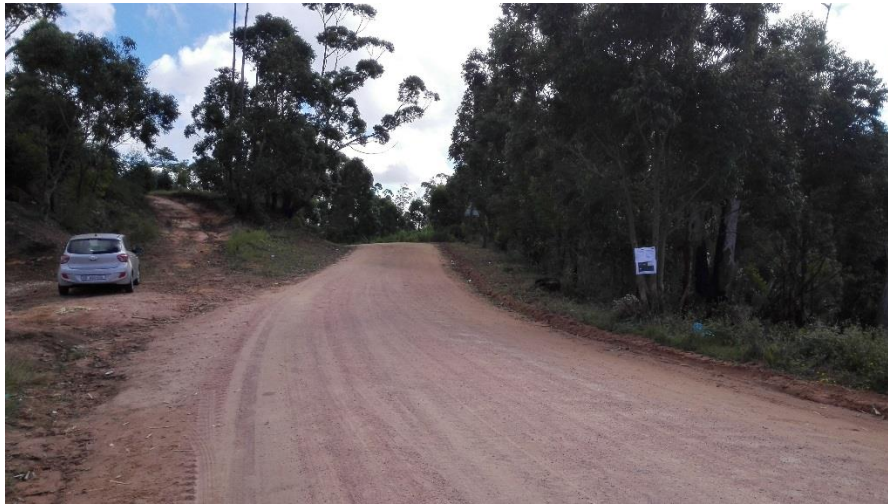
Photograph 1: Shows the existing condition of the start of the Nositha Road.
