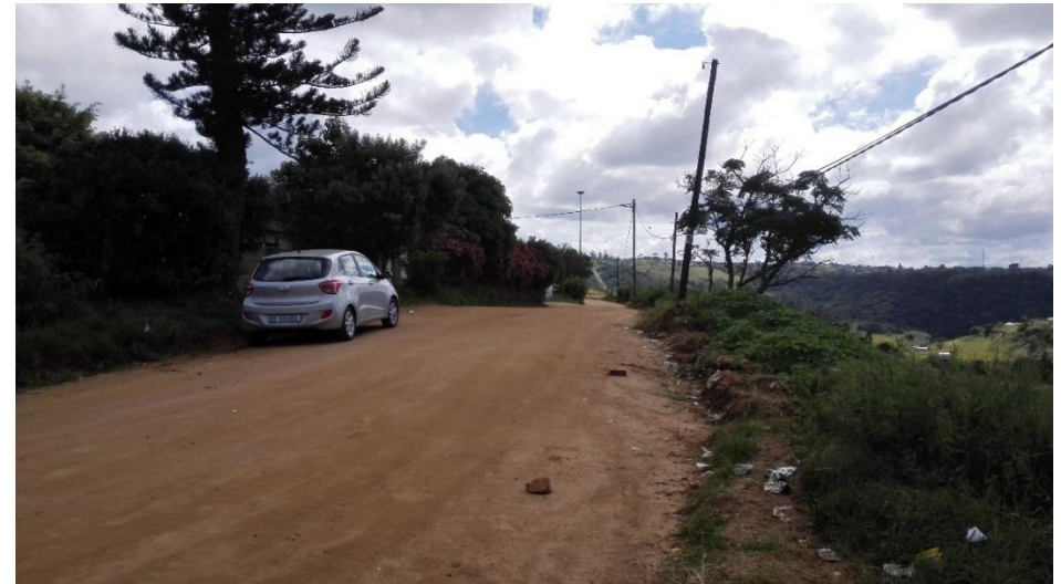
Photograph 6: Shows the existing condition of Nositha Road. Note, alien vegetation lines the road, and Eskom powerlines are in close proximity to the road reserve.
