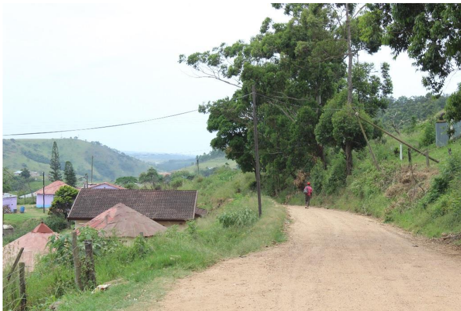
Photograph 3: Shows the existing condition of Nositha Road. Note, no storm water management system has been provided.
