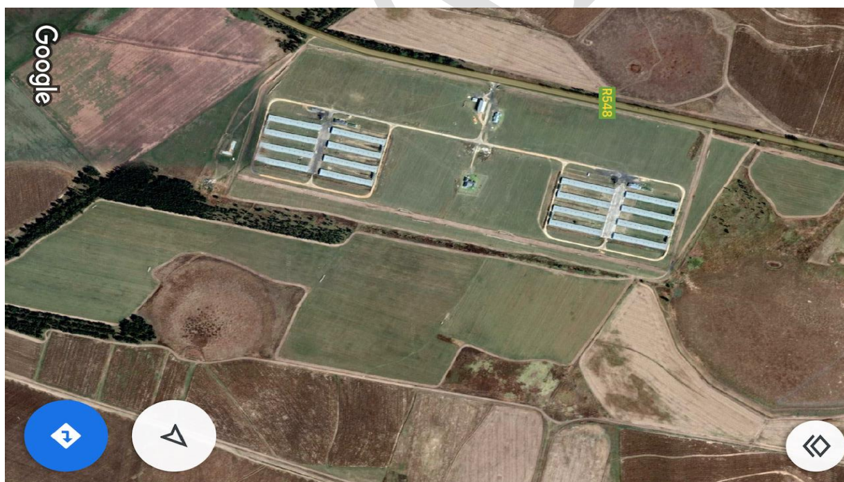
Figure 1: Image showing existing broiler houses on portion 17 of Modderbult 115IR
