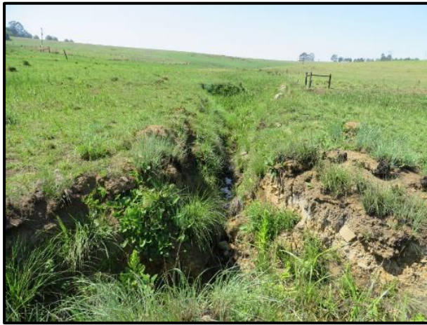
Plate 15. Excavated drain in Wetland Site 2. Erosion in the ditch is active.
