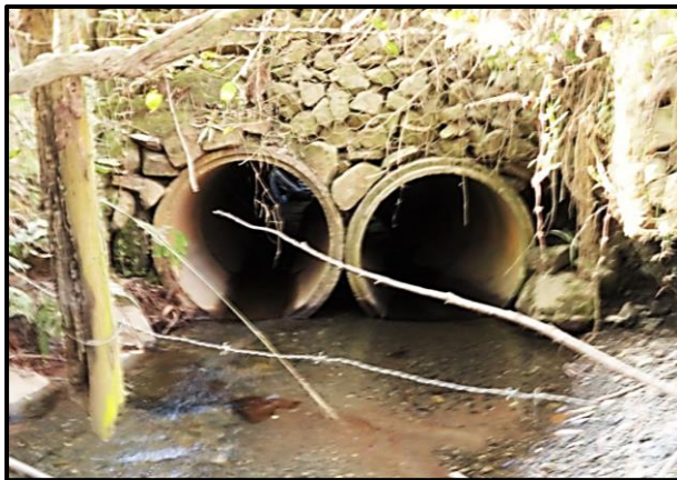
Plate 20. Road D494 stream crossing. Downstream end of the concrete pipes
