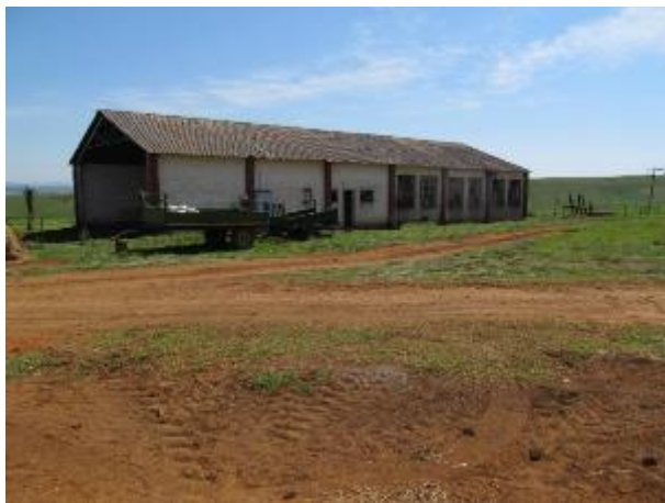
PLATE 1: Facing north at the old dairy site.
