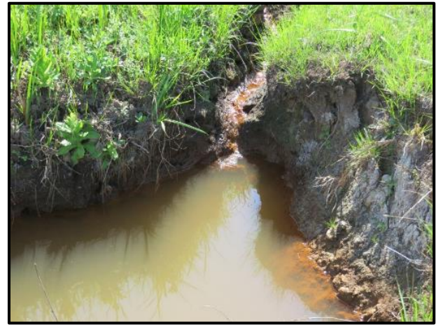
Plate 16. Active headcut erosion in a drainage ditch.
