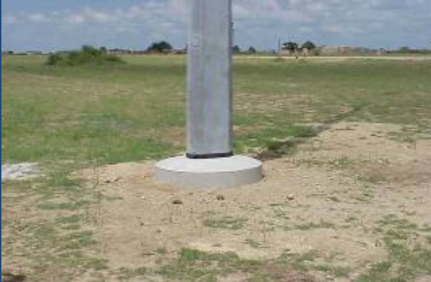
Figure 2: Pylon Excavation Foundation (source Eskom)
