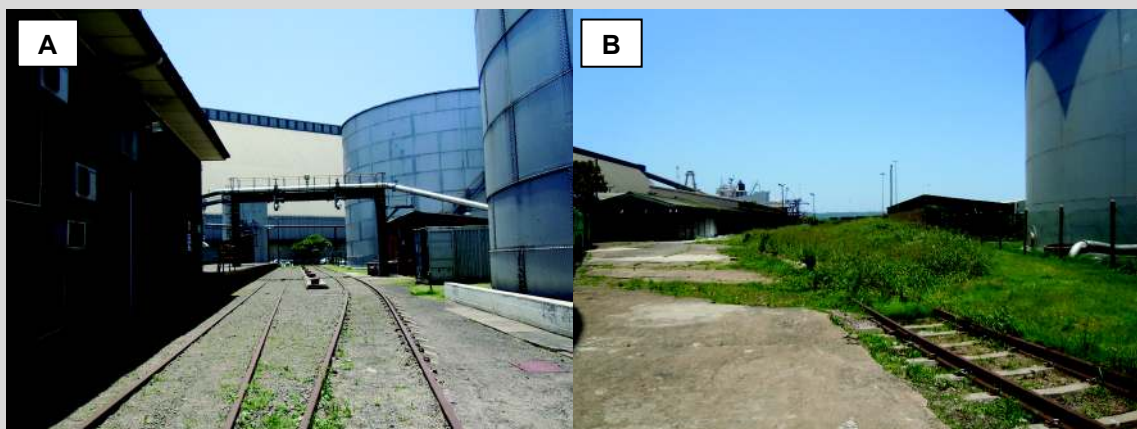
Figure 2: A) Disused Railway Track (i.e. Siding Number 650447) running through the main terminal site. B) Disused Railway Track dividing the Storage Terminal into two main portions.
