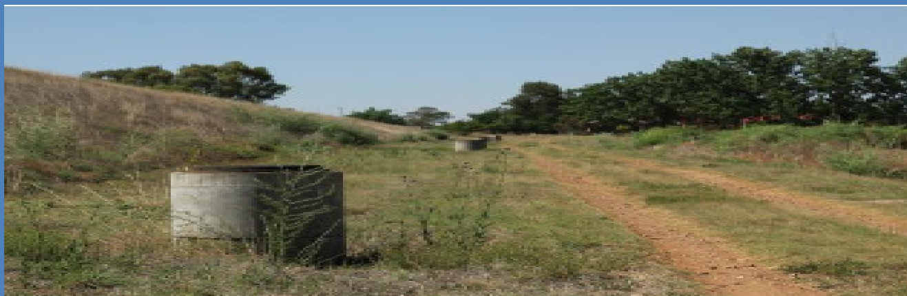
Figure 20: Row of Manholes.
