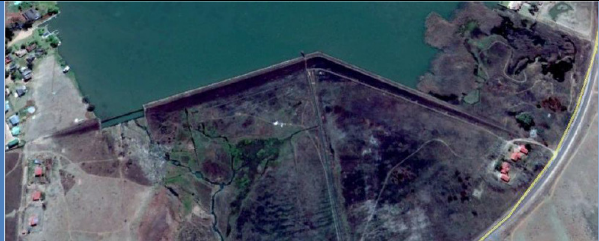
Figure 12: Rietspruit Dam Wall.
