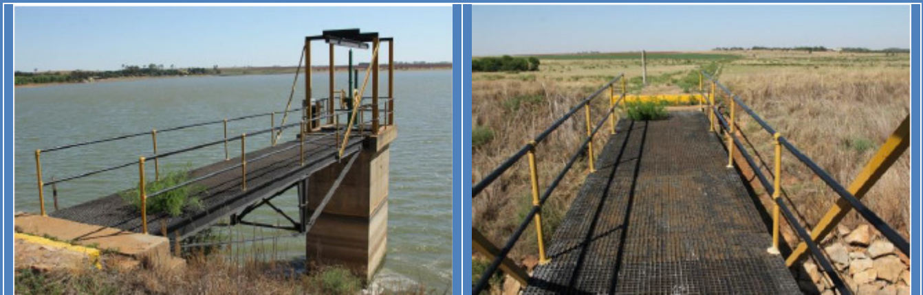
Figure 16: Outlet Tower and Access Bridge to the Outlet Tower.
