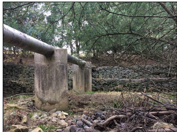
Plate 7-2: Existing Ø355mm steel pipeline at N3 crossing
