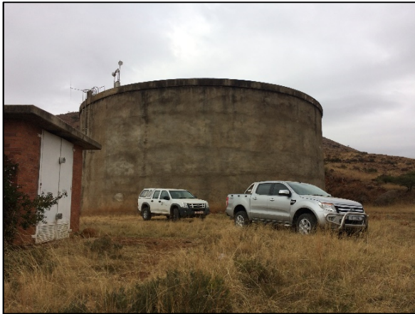
Plate 7-5: Existing 10MI Wembezi reservoir. New 10MI reservoir to be constructed adjacent to the existing reservoir
