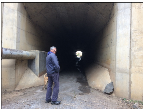
Plate 7-3: Existing Ø355mm steel pipeline at N3 culvert
