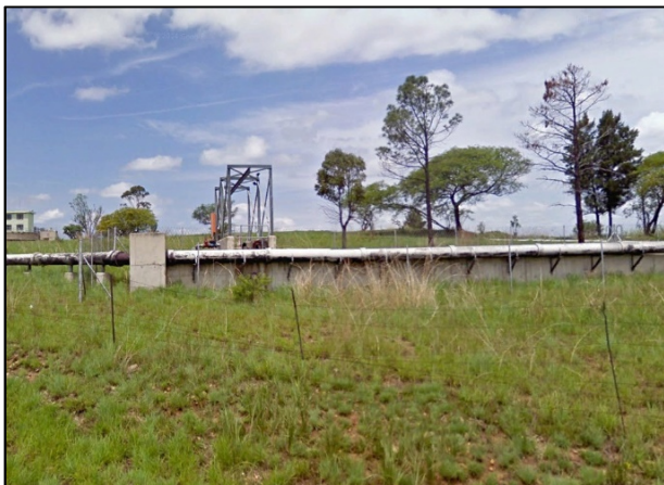
Plate 7-1: George Cross Water Treatment Works
