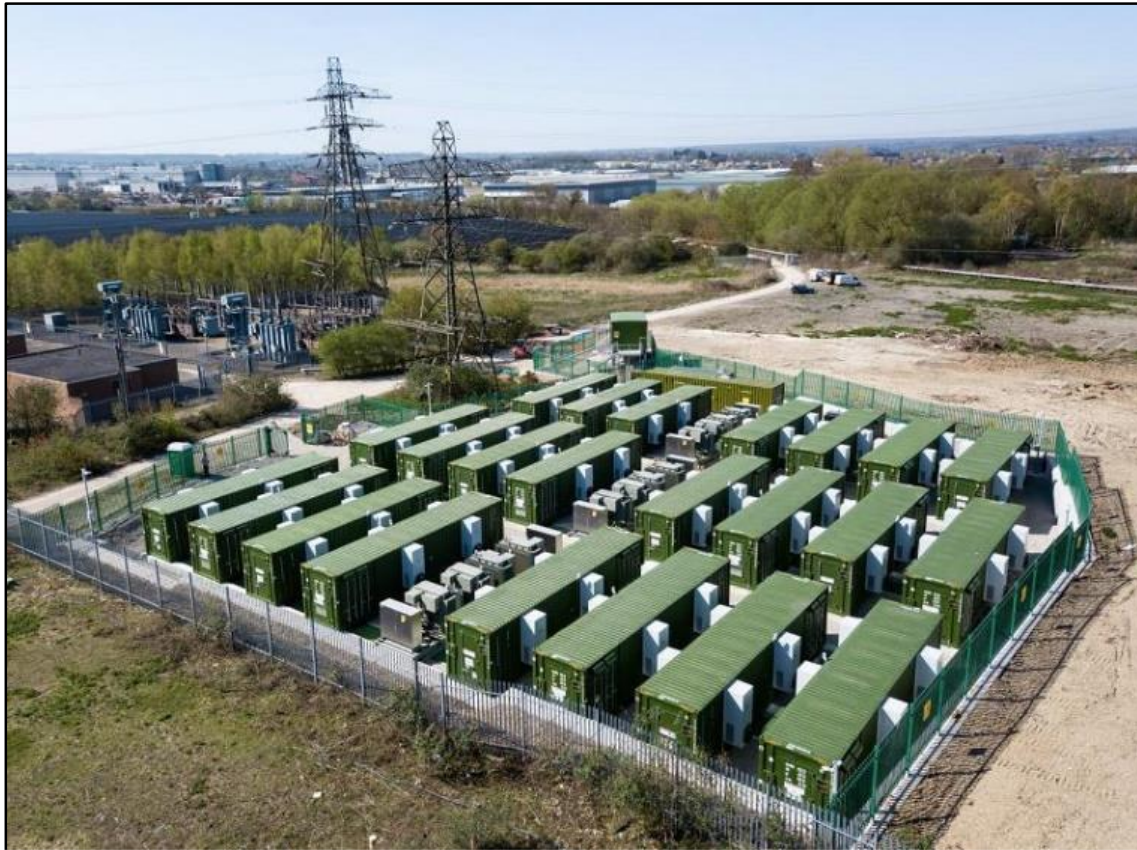
Figure 5: Example of a 29 MW BESS located in Aylesford, UK (Source: Eskom 2018)
