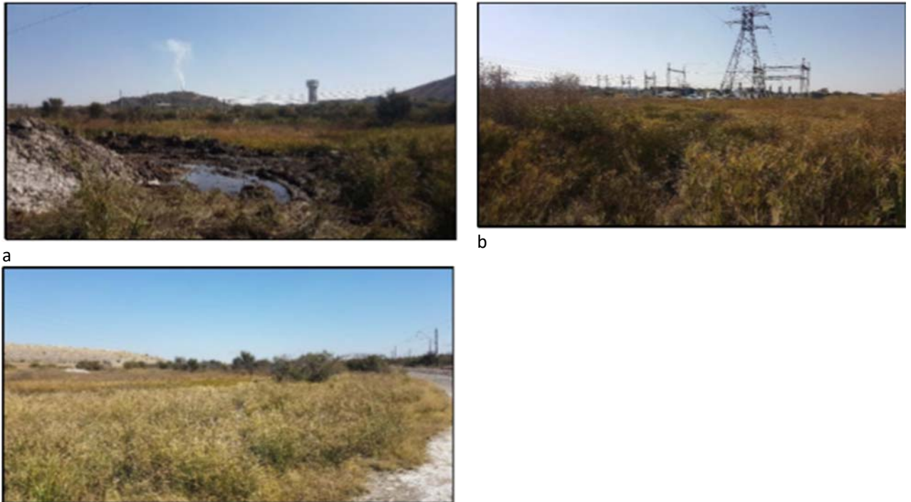
Figure 16: a. Excavation activities taking place within the artificial seep wetland, b. Wetland vegetation in the foreground, with the existing substation and overhead powerlines visible in the background, c. Wetland vegetation adjacent to the existing substation
