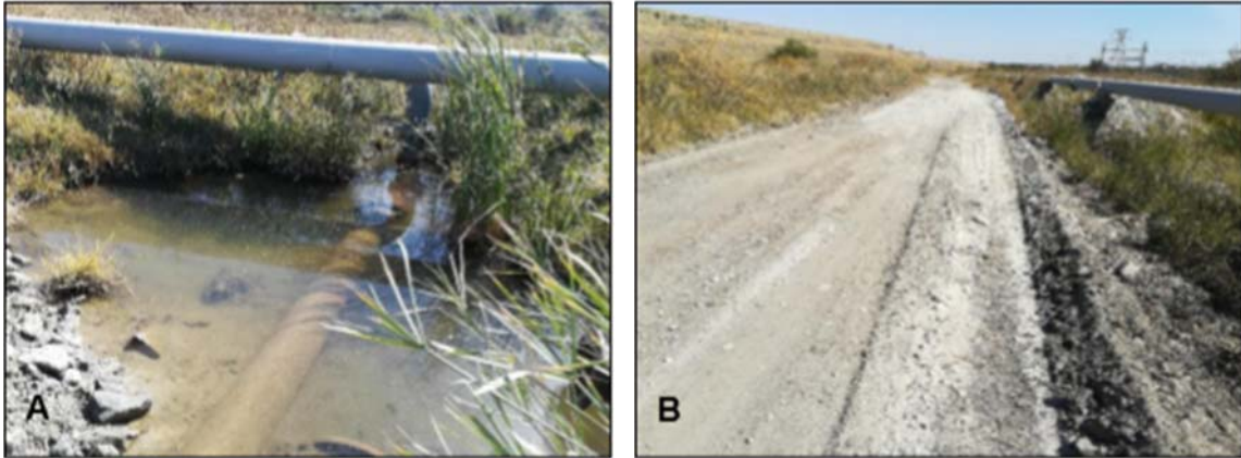
Figure 24: a. Pipelines found within the wetland, b. informal gravel roads that traverse the wetland
