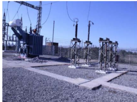
b. Existing transformer bay
