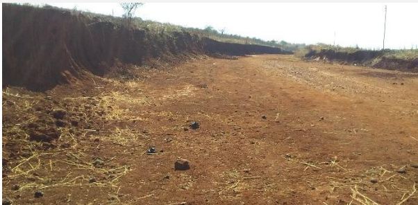
Trench on the entrance of the farm
