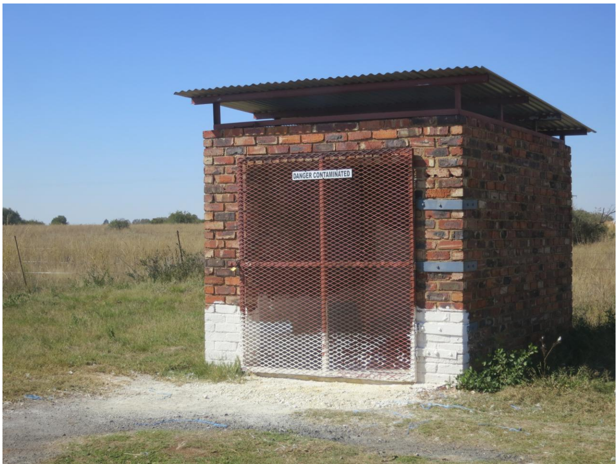
Figure 7: Example of a mortality room where mortalities are stored prior to daily collection
