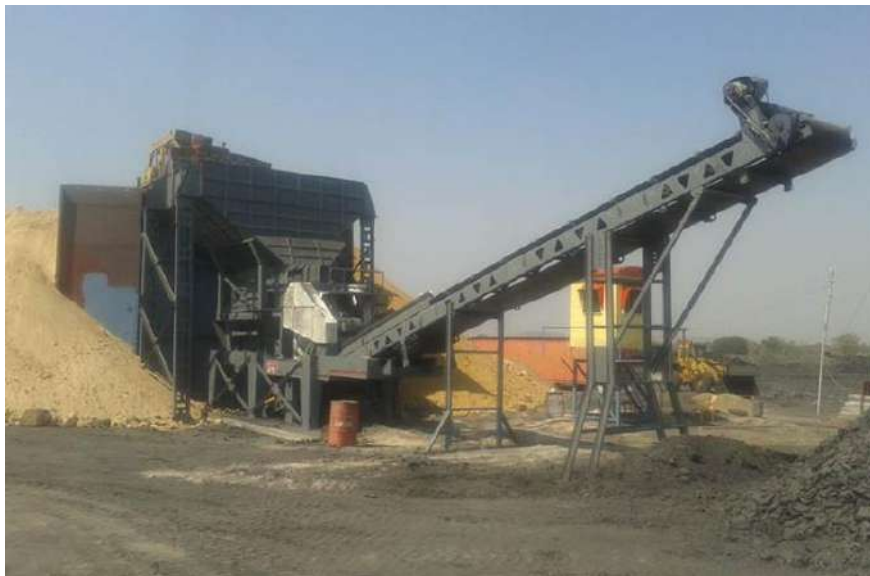
Figure 11: Typical example a coal crushing and screening unit.
