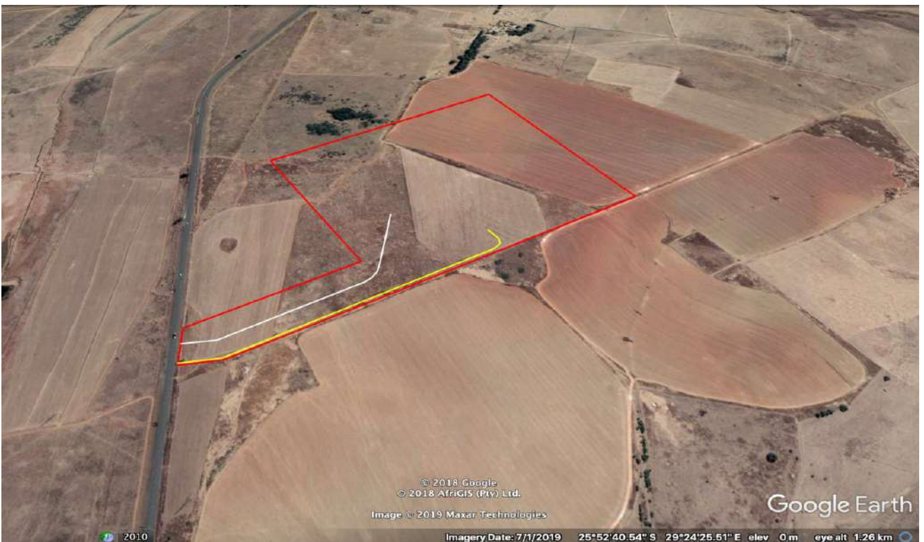
Figure 3 & 4: The Powerline will traverse from Silimela substation (top). The line will run through largely agricultural landscape bypassing farm settlements, villages and town settlement
