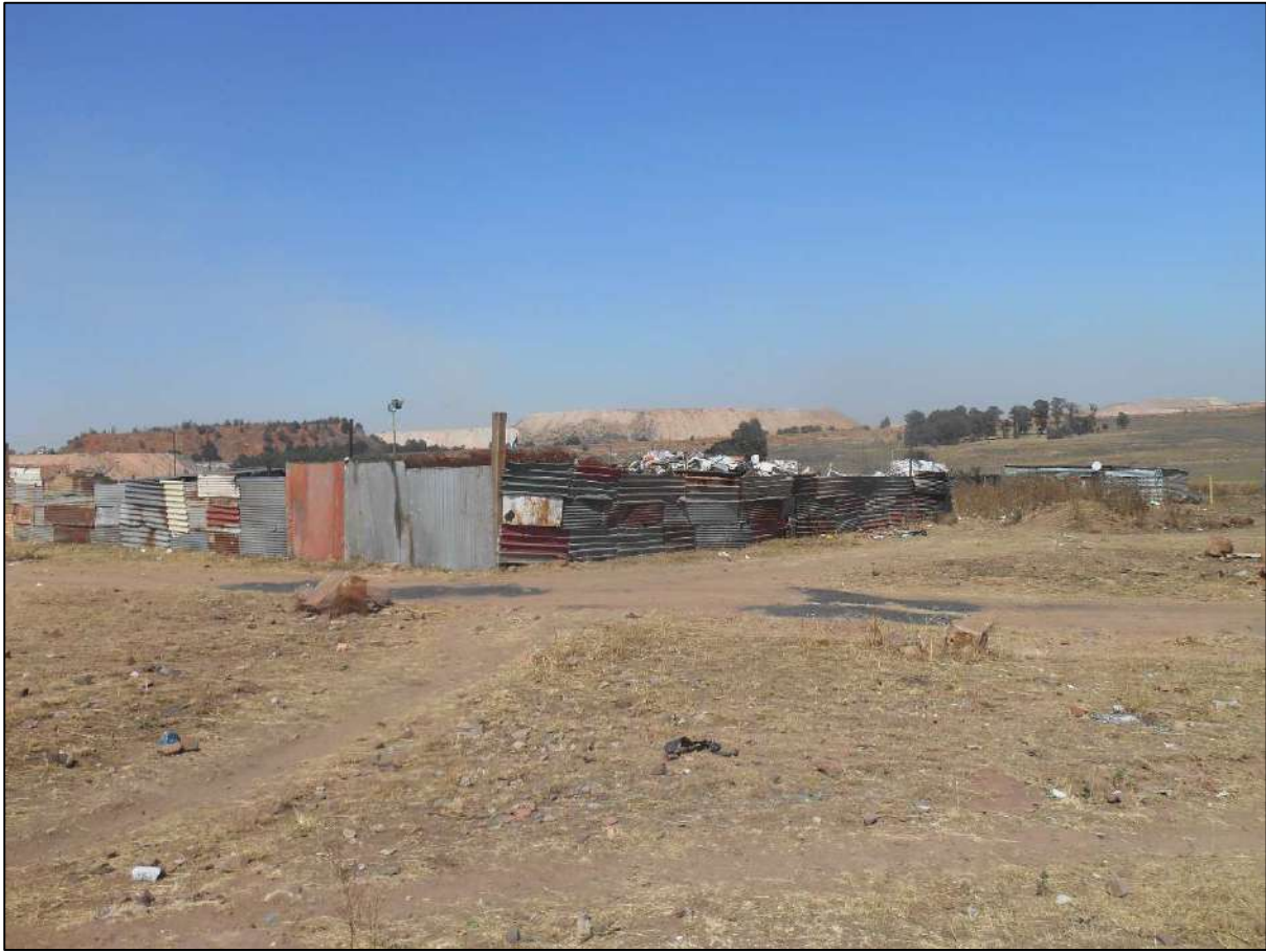
Figure 8: Affected Structure in Mhluzi
