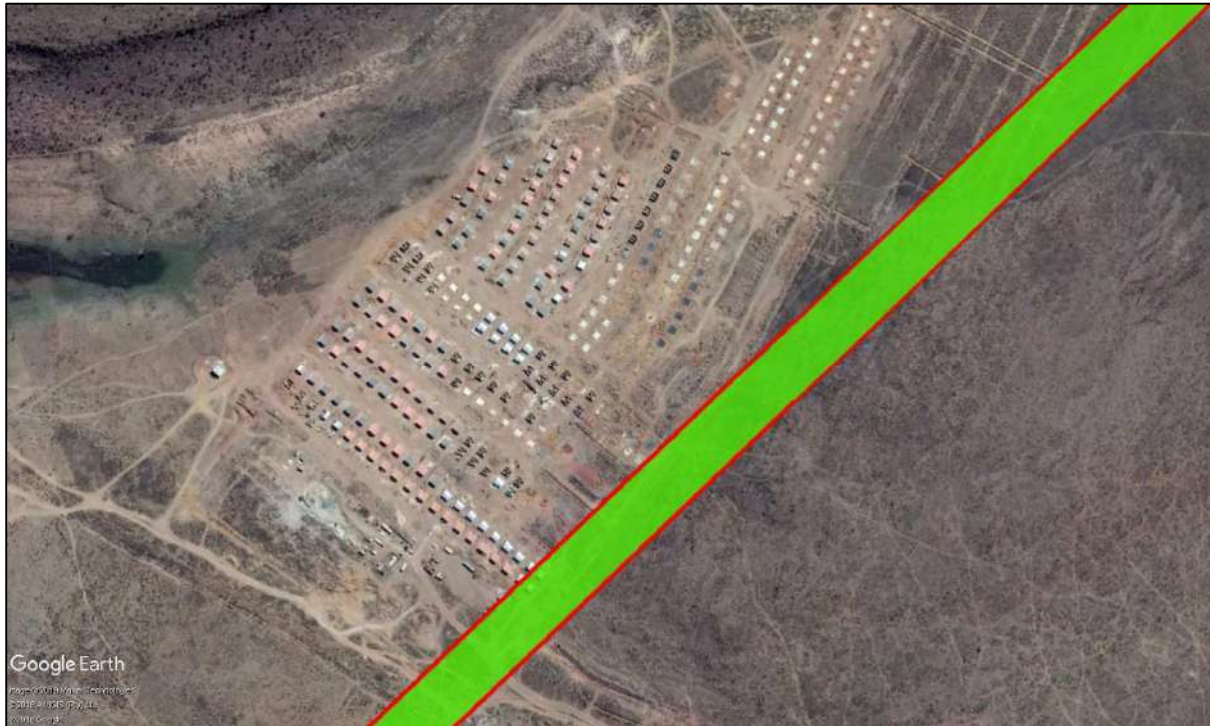
Figure 10: Impacted Structures in Mhluzi Ext 2 [25°44'13.77" S, 29°25'14.77" E]
