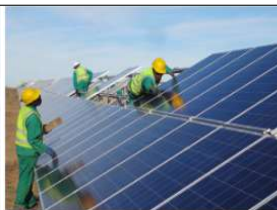
Figure 2.5: Picture of the installation of a typical PV array (75 MW plant in Kalkbutt South-Africa Source: PennEnergy)
