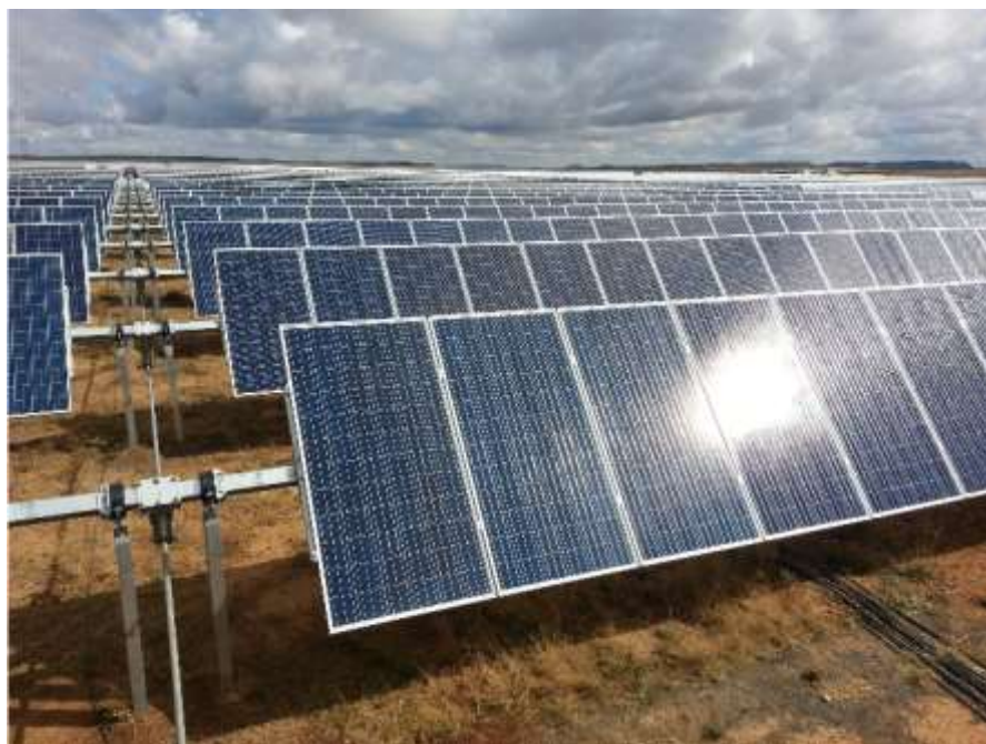
Figure 2.7: The support structures elevate the PV panels and allow for single axis tracking of the sun for increased efficiency (Source: SAPVIA)
