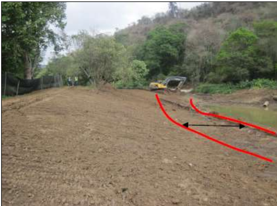
Figure 16: Example of the creation of a terrace on the dam fringe to allow for the establishment of wetland vegetation (Source: GroundTruth).
