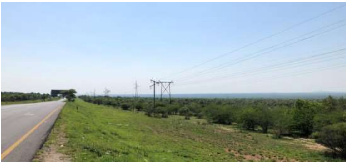
Figure 54: View looking east along the R556 road showing the existing power lines routed south of this road in contrast to the proposed routing of the power line linking the SEZ zone and the Ngwedi Substation north of this road.
