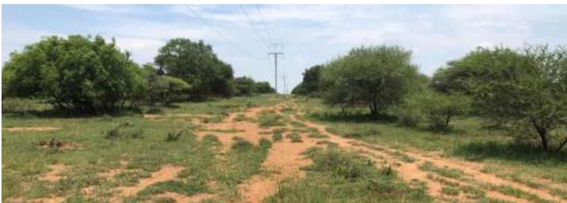
Figure 45: View of the existing power-line corridor linking the SEZ zone with the Ngwedi Substation at the east end of the corridor (southern edge of the SEZ zone).
