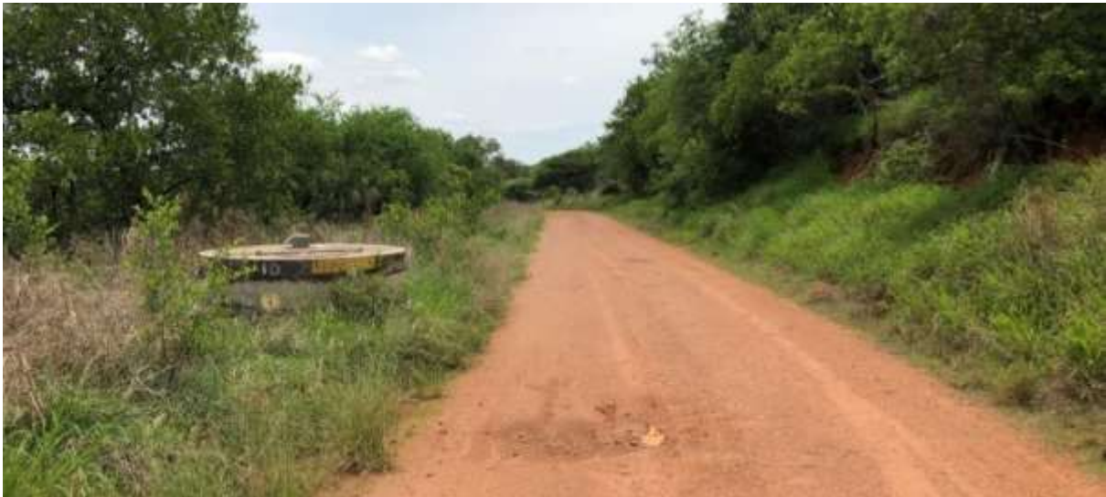
Figure 49. View of the existing water pipeline route which is proposed to be upgraded in the eastern portion of its route close to Vaalkop Dam.
