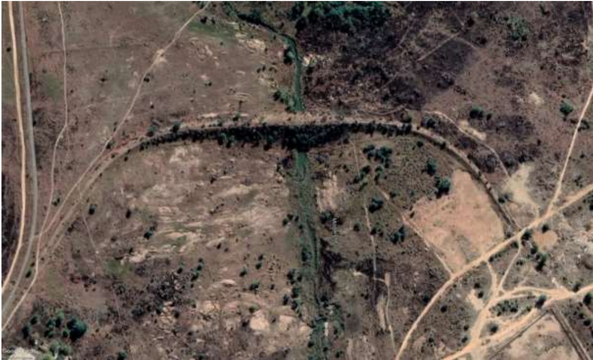
Figure 62: Section of the old railway line, showing the culvert crossing the Mogwase spruit
