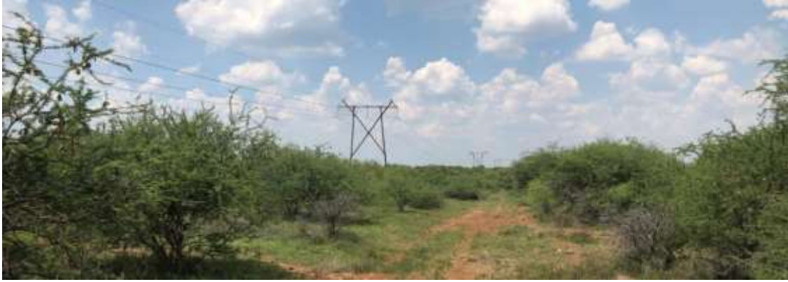
Figure 46: Another view of the existing power-line corridor in the middle reaches of the corridor linking the SEZ zone and Ngwedi Substation.
