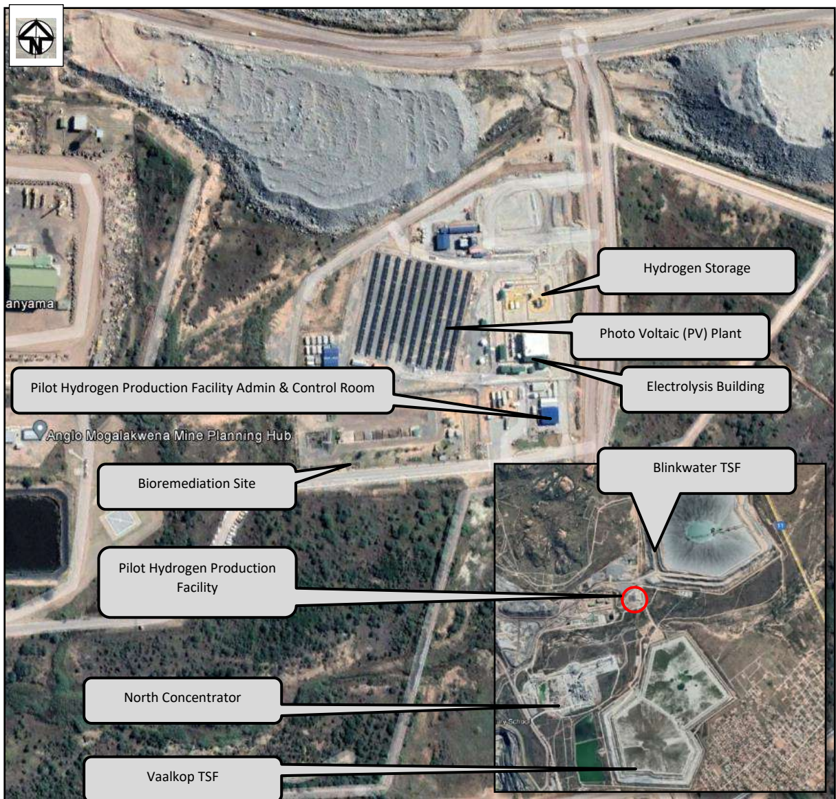
Figure 3-25: Existing Pilot Hydrogen Production Facility
