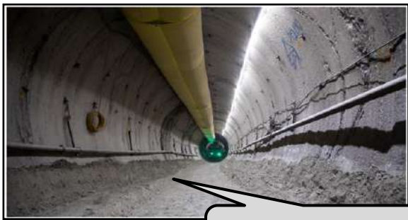
Mobile Tunnel Borer Machine
