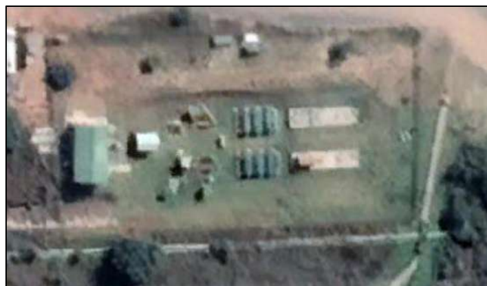
Figure 3-18: North Concentrator WWTW
