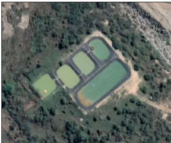
Figure 3-19: Image of the Contractors Camp WWTW
