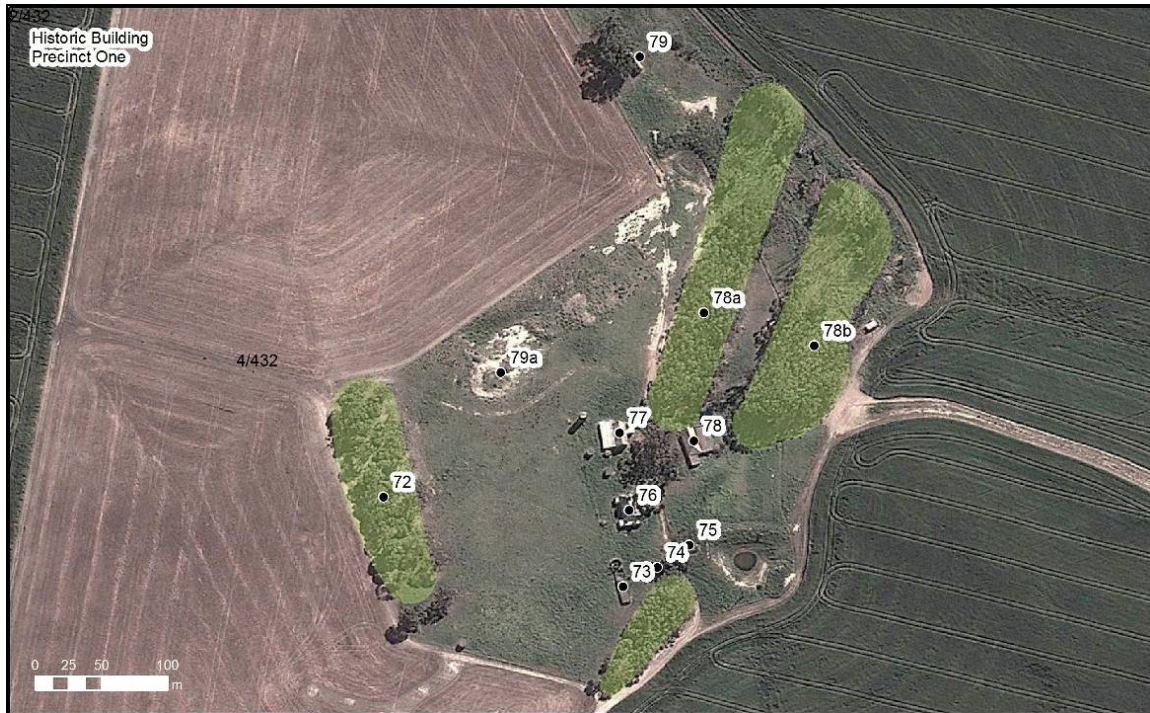
Figure 8. 20: Mapping of heritage resources in Historic Bldg Precinct One (Source: GoogleEarth)
