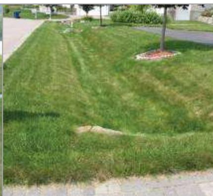
Figure 14: Grass lined channel
