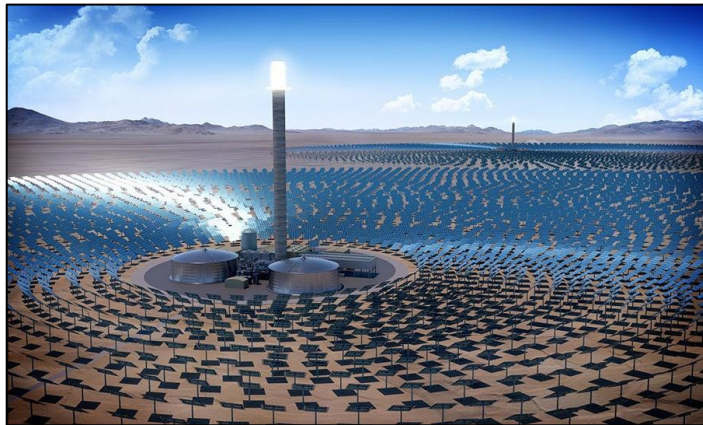
Figure 11 General appearance of a CSP solar plant.
