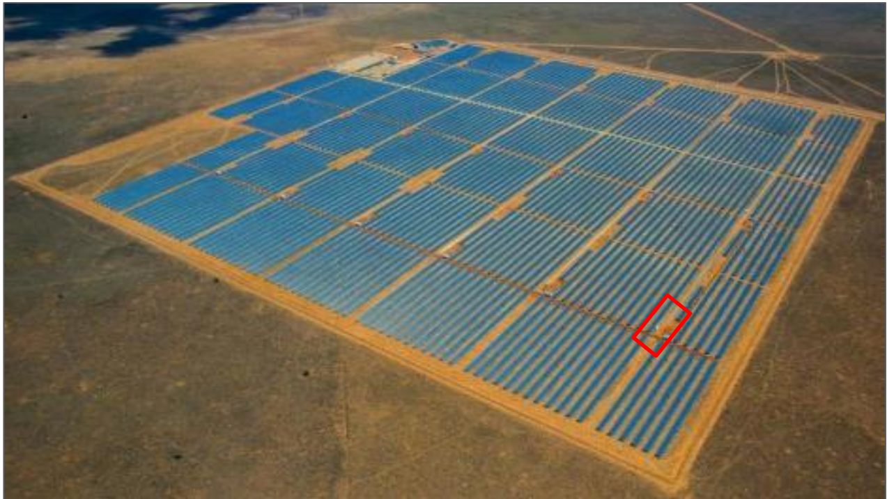
Figure 5-4: Inverter positioning on a PV panel array. The red block illustrates the location of an inverter within a PV panel array.
