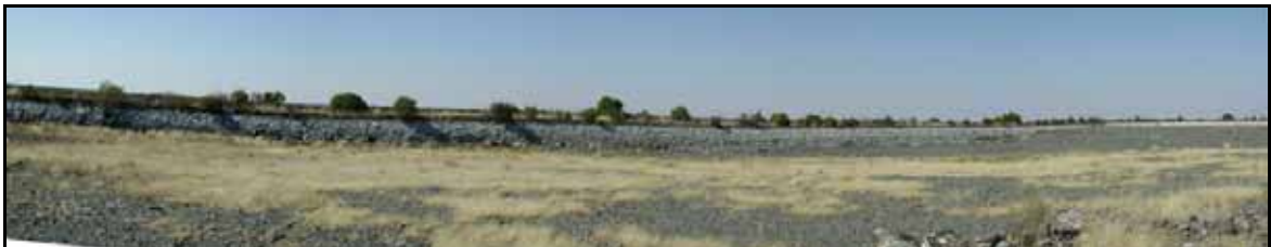
Figure 16: Dried-out return water dam at Pering Mine
