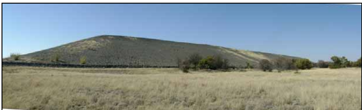
Figure 13: Tailings dam at Pering Mine
