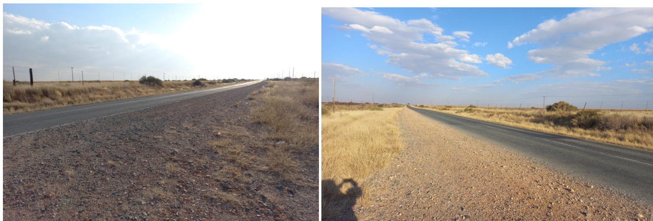
FIGURE 45: THE ENTRANCE OF THE R3112 ROAD AT SITE B – LINE OF SIGHT IS GOOD IN BOTH DIRECTIONS.
