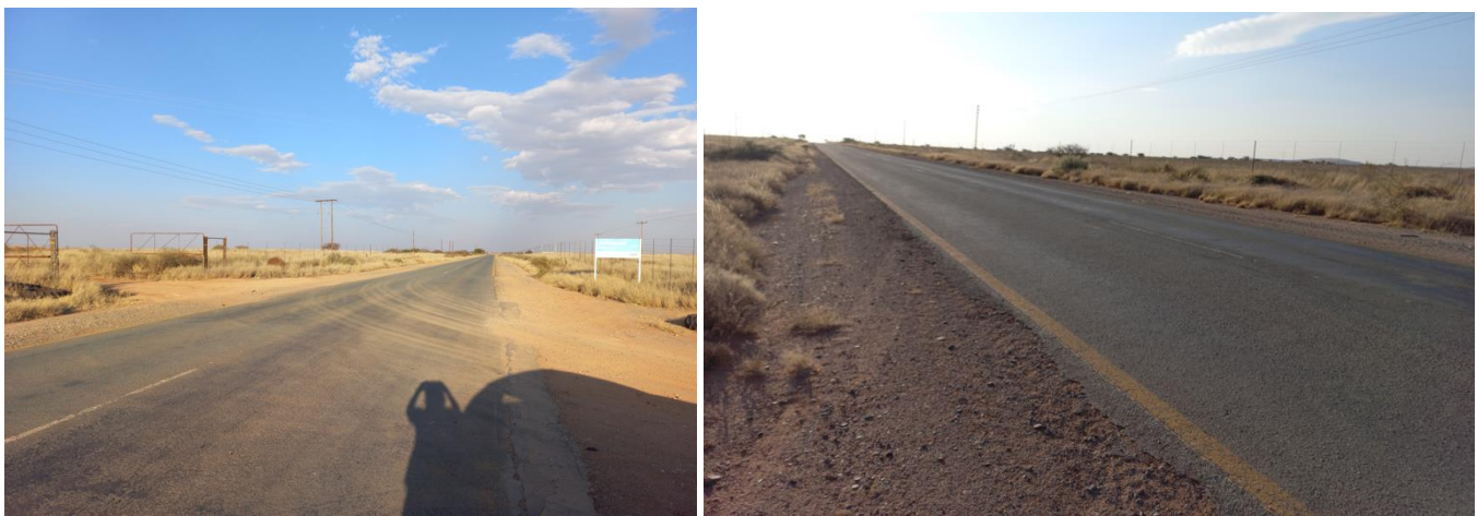
FIGURE 44: THE ENTRANCE OF THE R3112 ROAD AT SITE A – LINE OF SIGHT IS GOOD IN BOTH DIRECTIONS.
