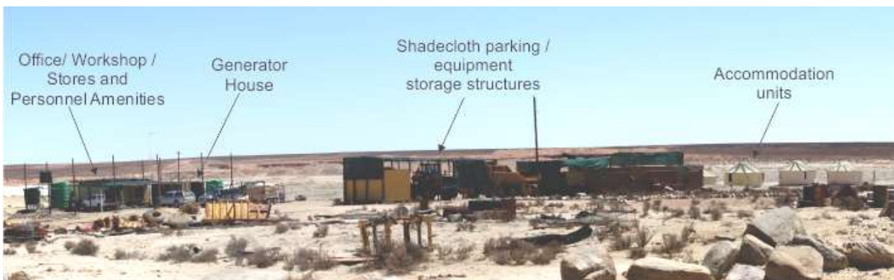
Photo 3: Status of facilities at Bosluispan looking west
