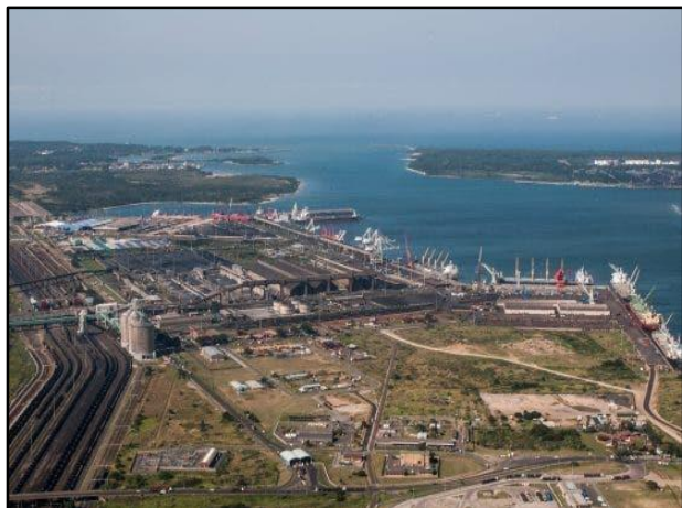
Figure 0-1: Overview of the Port of Richards Bay
