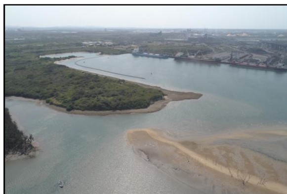
Figure 0-1: Overview of Port Site
