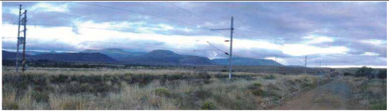
Figure 10.7 View of Infrastructure including Railway Line, Drennan substation and associated Powerlines
