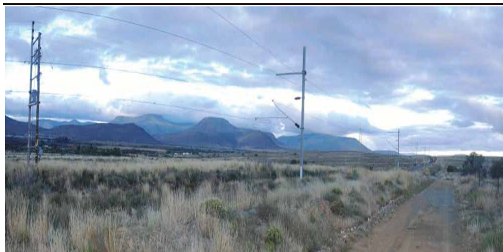
Figure 6.10 View of the Project Site showing existing railway line
