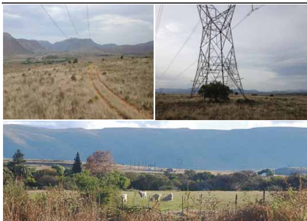
Figure 10.12 Overhead transmission lines and Drennan substation at the Site
