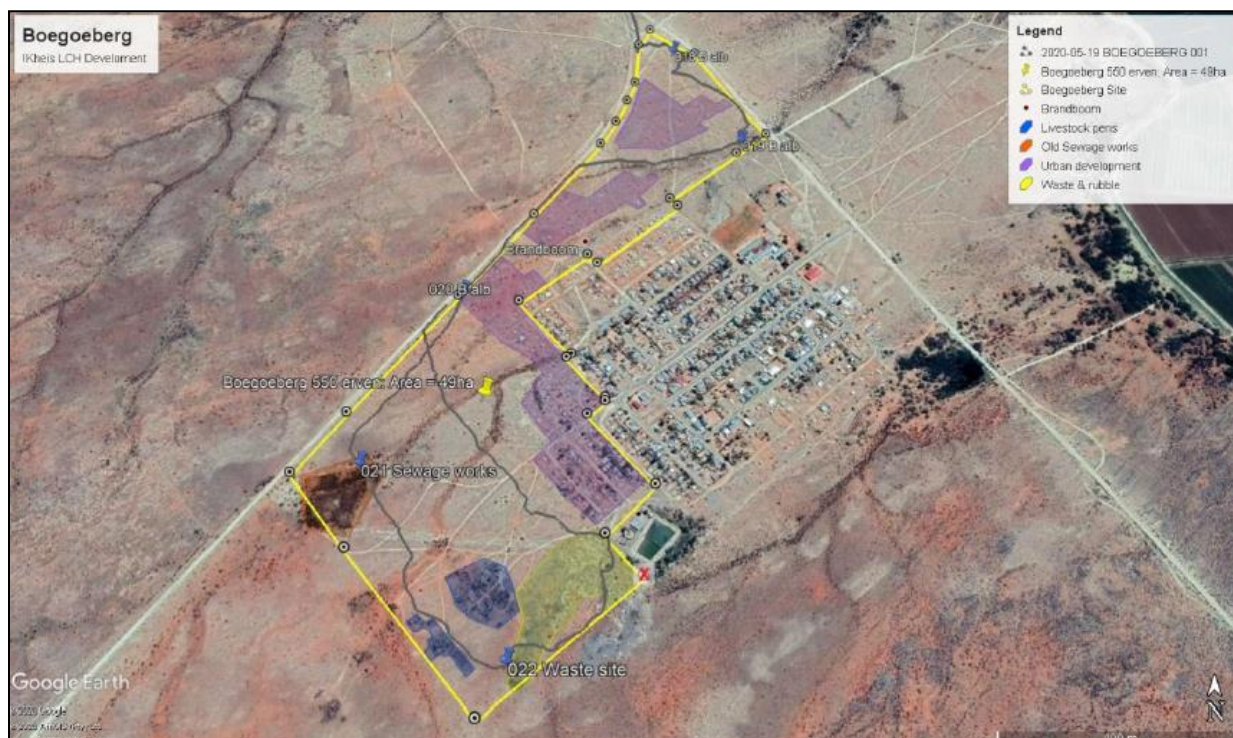
Figure 25. Overview of the site, showing most significant disturbed areas (Source: Botanical Impact Assessment, Appendix 6A)
