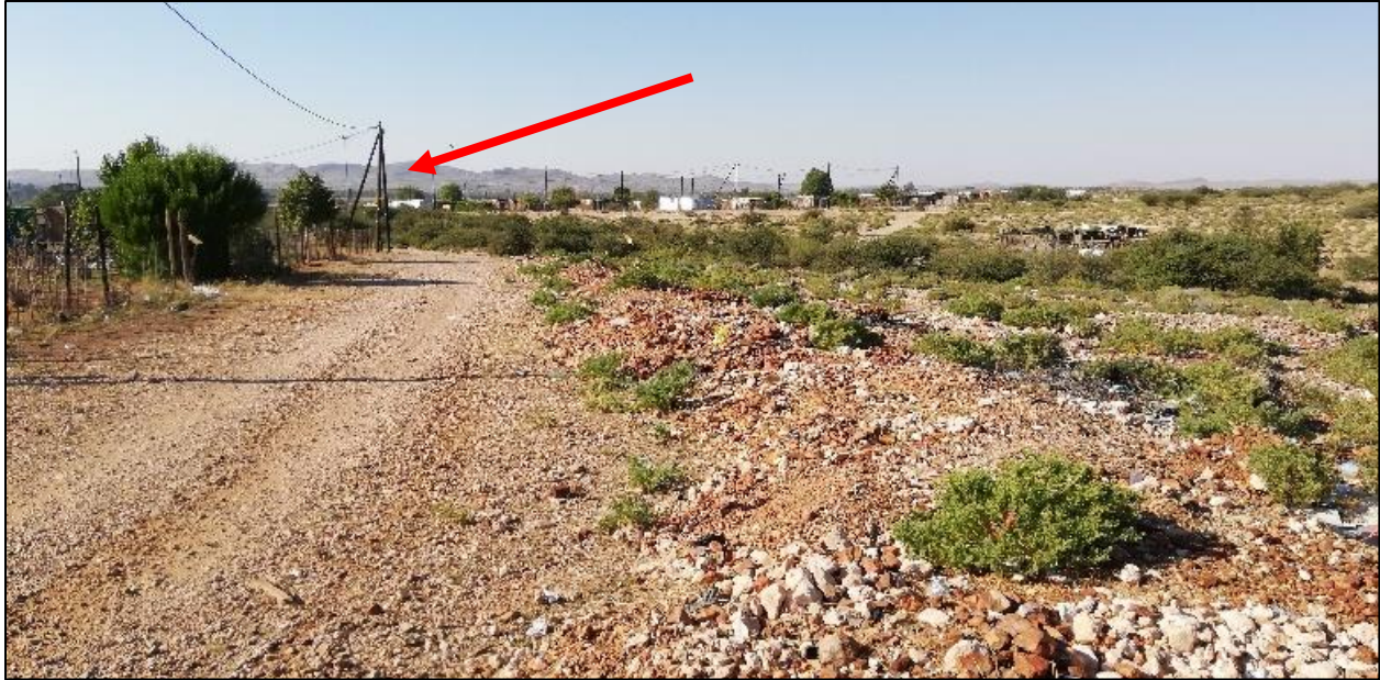
Figure 10. Overview of site looking in a south-east over the site. Note existing electrical supply (red arrow).
