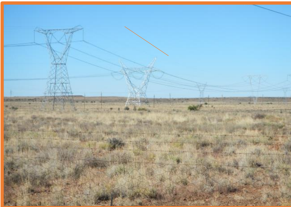
Figure 16 &17: Existing transmission lines near the Droërvier Substation.
