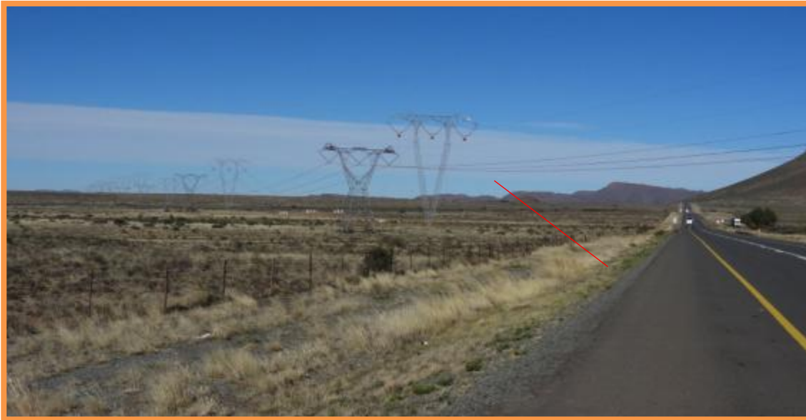
Figure 15: View of the existing power line crossing the N1 main road.
